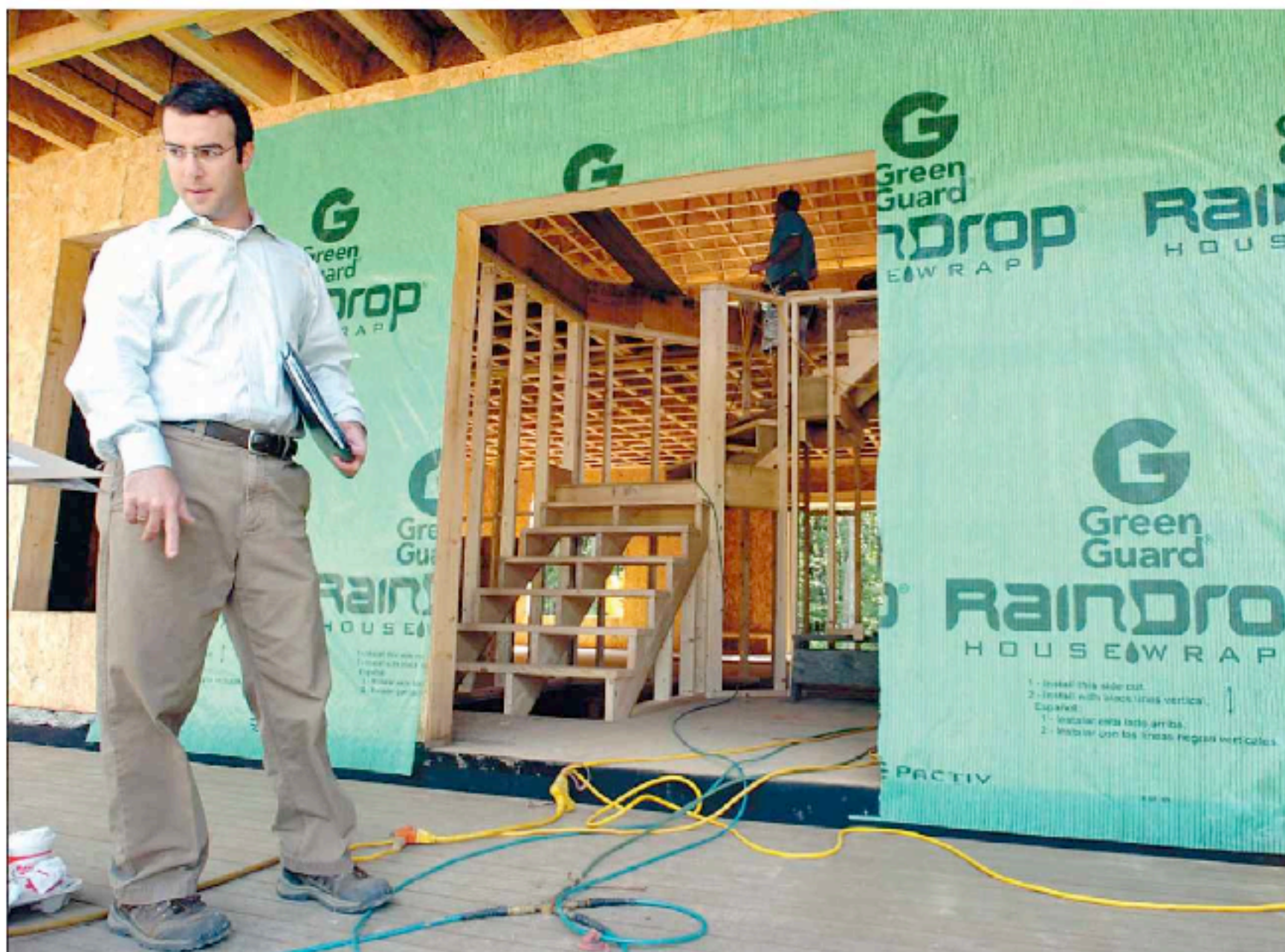
Developer Joe Samra points out the different green features like the Green Guard RainDrop Housewrap, which has drainage channels to move water away from the wall.
